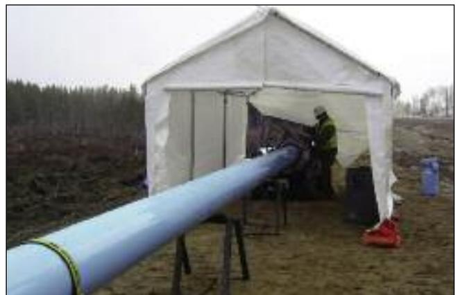
*The shelter of a tent combined with the heat from the fusion machine was enough to keep the pipe ends at the required temperature for fusing.*
